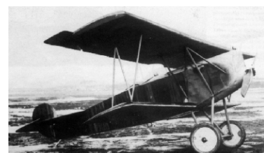
Fokker V 11/II, although with the same w/n 1883 as V 11/I, the significant changes are clearly visible. This plane took part on the Adlershof Fighter competition. (Albatros/PL Gray Collection-used with permission)
