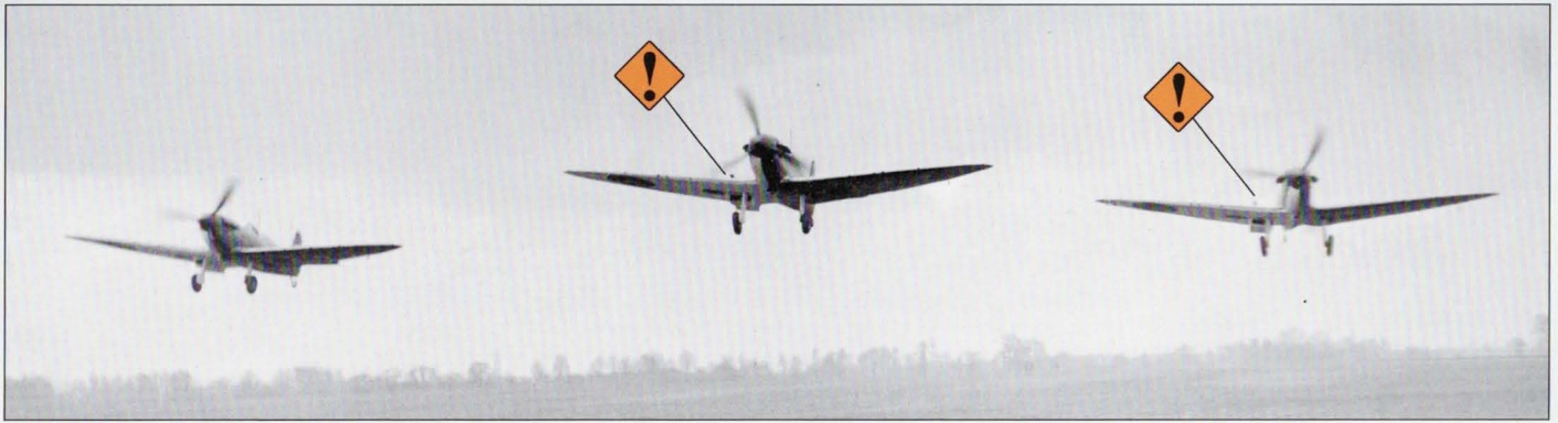
Unidentified early production Spitfire Mk.I fitted with DH.5/39 propellers take off for a training flight sometime after late April 1939. Note the repainted white and Night undersides with subdued B Type roundels and the Williamson G.22 camera guns mounted on their starboard wings.
