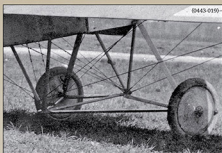
Undercarriage detail from Fokker E.II 36/15 showing strut fairings and rigging details.
