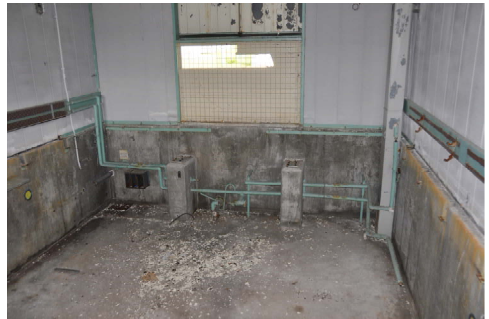
Below, a view into the pit. Note the columns at the back which supported the launcher and above them, the blow-out panel.
