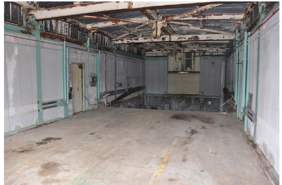
Above, a view inside the decommissioned shelter. Note the pit in the back of the shelter. The area around the launcher was covered with a steel grating.
