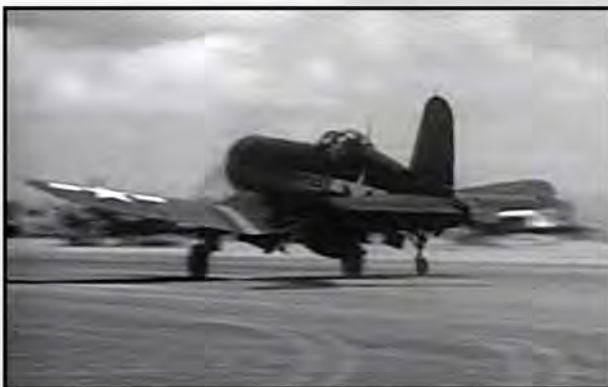
Three frames from a motion picture that show the unusual markings carried by 57522. Note the Neutral Gray 43 (?) 165 gallon Lockheed drop tank, the lack of a tail hook in the hook well, and the small aerodynamic fairing aft of the tail wheel.
