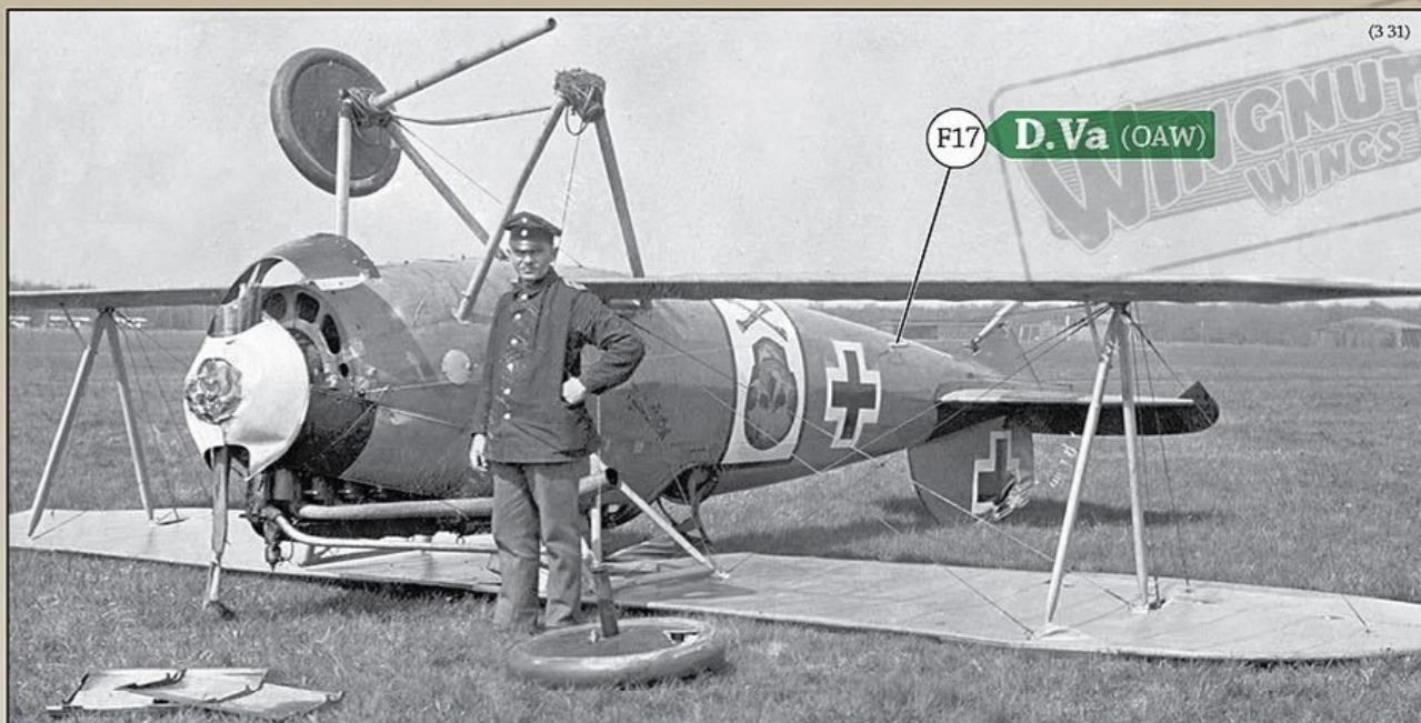
A mechanic poses in front of Hans von Goessel's crashed OAW built Albatros D.Va, the two undercarriage axle wing fairings at the bottom left of the photo possibly indicating the start of his salvage mission. Note the aileron control wires entering the upper wing, undercarriage bungee cords and OAW style lifting handle 'bar' protruding from the rear side of the fuselage. The name under the cockpit opening reads 'Margarethe'.
